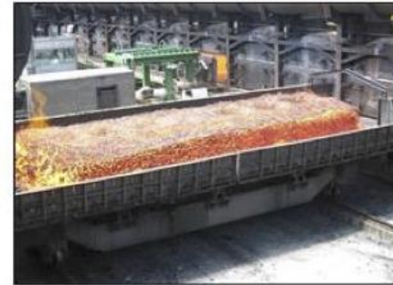
Heat Recovery (HR-CO)
